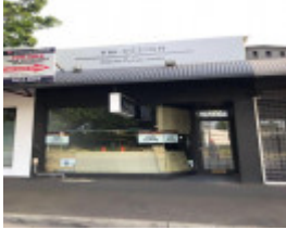
119 Station Street, Malvern
