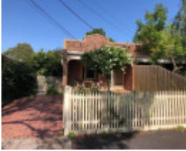
36 Victoria Road North, Malvern
