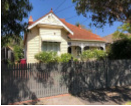
42 Victoria Road North, Malvern
