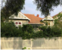
45 Victoria Road North, Malvern
