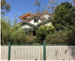
48 Victoria Road North, Malvern
