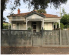
55 Victoria Road North, Malvern
