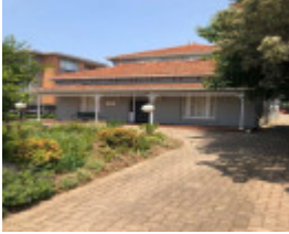
170 Wattletree Road, Malvern
