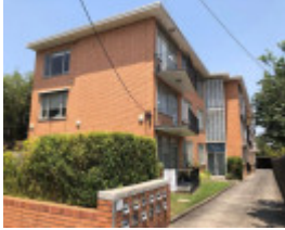
172 Wattletree Road, Malvern
