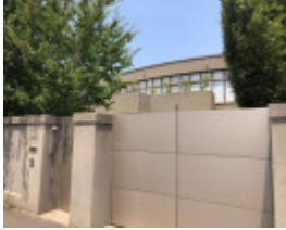
174 Wattletree Road, Malvern
