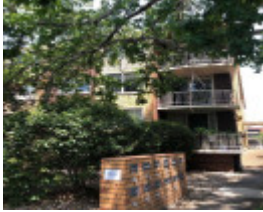
184 Wattletree Road, Malvern
