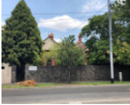
198 Wattletree Road, Malvern
