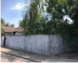
224 Wattletree Road, Malvern
