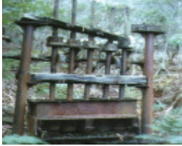
1 pioneer battery site pioneer creek bonang front view
