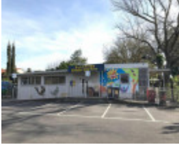
5 Cooinda Place, Malvern East
