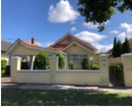
1157 Dandenong Road, Malvern East
