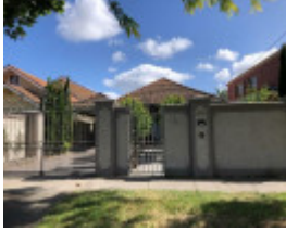
1159 Dandenong Road, Malvern East
