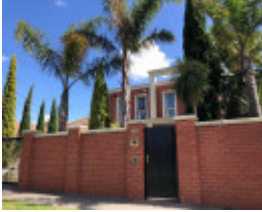
1161 Dandenong Road, Malvern East
