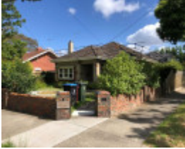
1173 Dandenong Road, Malvern East
