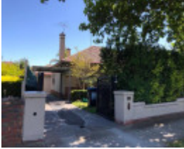
1179 Dandenong Road, Malvern East
