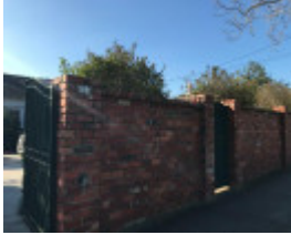
1191 Dandenong Road, Malvern East
