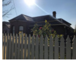
1201 Dandenong Road, Malvern East
