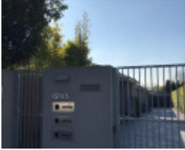
1205 Dandenong Road, Malvern East
