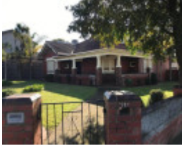
1213 Dandenong Road, Malvern East
