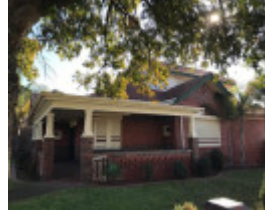
1213 Dandenong Road, Malvern East
