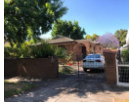
4 Fountaine Avenue, Malvern East
