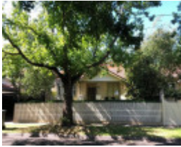
18 Fountaine Avenue, Malvern East
