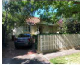
18 Fountaine Avenue, Malvern East
