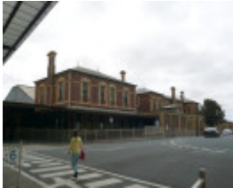
GEELONG RAILWAY STATION SOHE 2008
