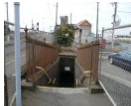
GEELONG RAILWAY STATION SOHE 2008
