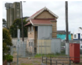
GEELONG RAILWAY STATION SOHE 2008
