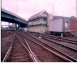
Geelong Railway Station Signal Box
