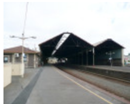
GEELONG RAILWAY STATION SOHE 2008
