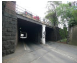
GEELONG RAILWAY STATION SOHE 2008
