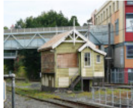
GEELONG RAILWAY STATION SOHE 2008
