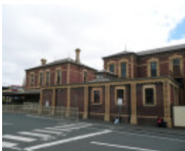
GEELONG RAILWAY STATION SOHE 2008
