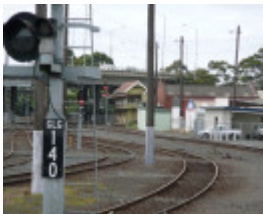
GEELONG RAILWAY STATION SOHE 2008
