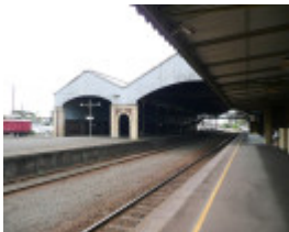
GEELONG RAILWAY STATION SOHE 2008
