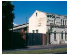
h01810 4 Melbourne omnibus building 1997
