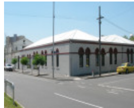
FORMER MELBOURNE OMNIBUS COMPANY'S STABLES SOHE 2008
