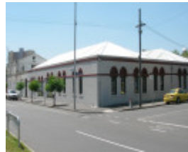
FORMER MELBOURNE OMNIBUS COMPANYS STABLES SOHE 2008
