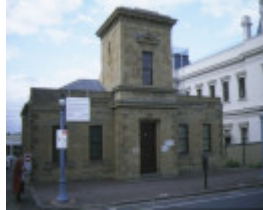
1 former telegraph station ryrie street geelong front elevation apr1997
