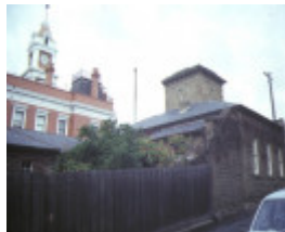
former telegraph station ryrie street geelong rear view jul1984
