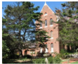
Wardell Building from nth west.jpg
