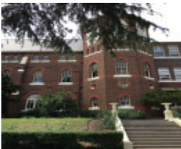
west side of Wardell Bldg.jpg
