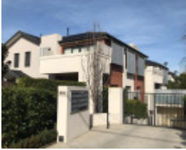
410 Waverley Road, Malvern East
