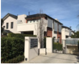
410 Waverley Road, Malvern East
