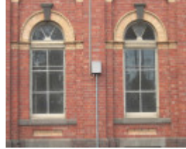
GAS REGULATING HOUSE SOHE 2008
