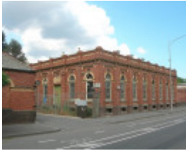
GAS REGULATING HOUSE SOHE 2008
