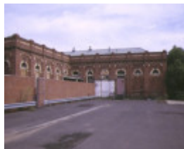
1 gas regulating house macaulay road north melbourne rear view apr1998
