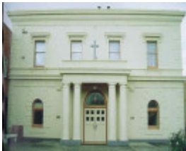
st johns lutheran church yarra street geelong front elevation publication
