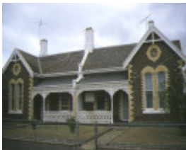
austin hall & terrace complex yarra & mundy streets south geelong terrace complex apr1997
