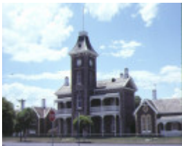
austin hall & terrace complex yarra & mundy streets south geelong front view of austin hall jan1997
