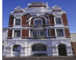
1 former royal hotel nelson place williamstown front view sep1998
