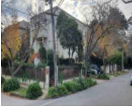
25 Glen Road, Toorak
