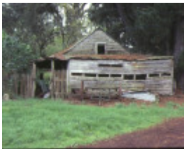
silverwells gembrook former post office & store
