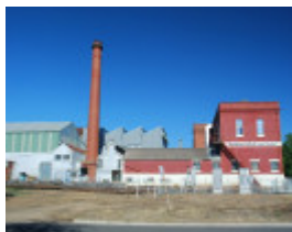
THOMPSONS KELLY & LEWIS ENGINEERING WORKS SOHE 2008
