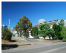
THOMPSONS KELLY & LEWIS ENGINEERING WORKS SOHE 2008
