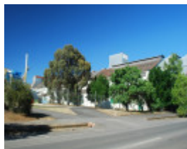
THOMPSONS KELLY & LEWIS ENGINEERING WORKS SOHE 2008
