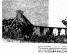
18.10 - Barton Hill Residence 01 - Shire of Whittlesea Heritage Study 1991
