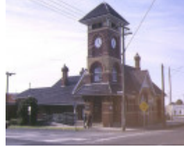
1 terang post office terang front view aug1998
