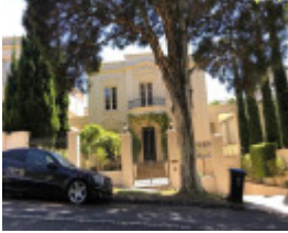
3B Glyndebourne Avenue, Toorak
