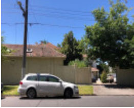
226 Kooyong Road, Toorak
