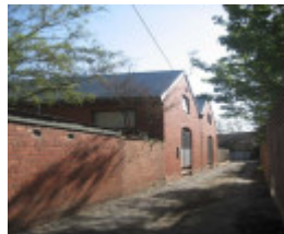
Brick warehouse at 9 Meryl Street.
