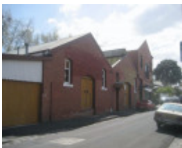
Edwardian brick warehouse at 5 to 7 Stuart Street.
