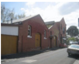
Edwardian brick warehouse at 5 to 7 Stuart Street.
