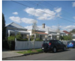
Victorian timber cottages on the north side of Barkly Avenue.
