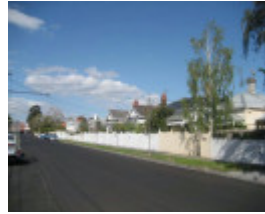
Victorian and Edwardian timber housing on the south side of Barkly Avenue.
