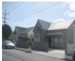
Victorian timber villa pair at 17 and 19 Stanhope Street.
