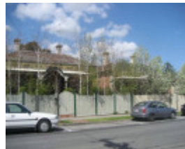
Victorian villas at 40 and 42 Lambeth Avenue.
