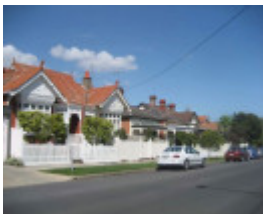
Edwardian and Victorian housing on the east side of Seymour Street.
