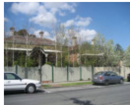
Victorian villas at 40 and 42 Lambeth Avenue.
