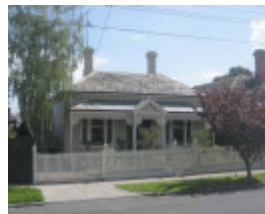
Victorian timber villa at 21 Seymour Avenue.
