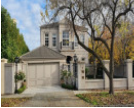
9 Power Avenue, TOORAK
