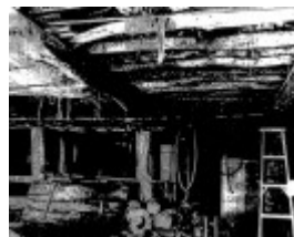
12.11 - Tregowan Cottage 10 - Shire of Whittlesea Heritage Study 1991
