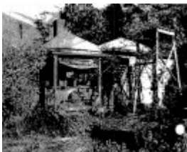
12.11 - Tregowan Cottage 06 - Shire of Whittlesea Heritage Study 1991
