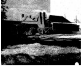
12.11 - Tregowan Cottage - Shire of Whittlesea Heritage Study 1991
