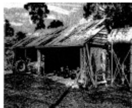
12.11 - Tregowan Cottage 08 - Shire of Whittlesea Heritage Study 1991
