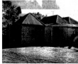
12.11 - Tregowan Cottage 02 - Shire of Whittlesea Heritage Study 1991
