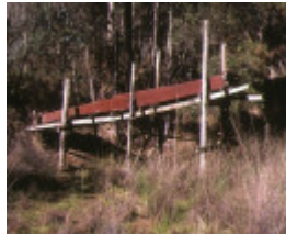
1 yackandandah creek gold hydraulic sluicing works yackandandah trestle side view mat1998
