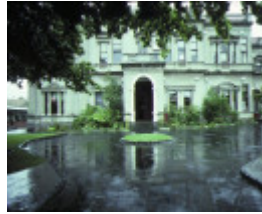
malvern house willoby ave glen iris entrance detail nov1985
