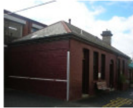
2017_Former laundry building.jpg
