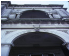
malvern house willoby ave glen iris arch detail aug1981
