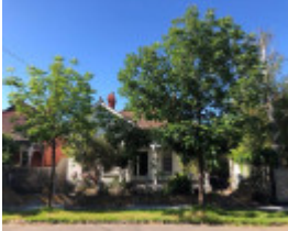
6 Alleyne Avenue, Armadale
