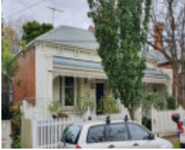
9-11 Hume Street, Armadale
