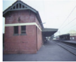
1 glenferrie railway station hawthorn station building jun1984
