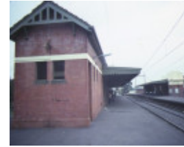
1 glenferrie railway station hawthorn station building jun1984
