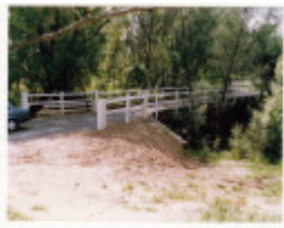
Timber Trestle Road Bridge over Diamond Creek Colour 1 - Shire of Eltham Heritage Study 1992
